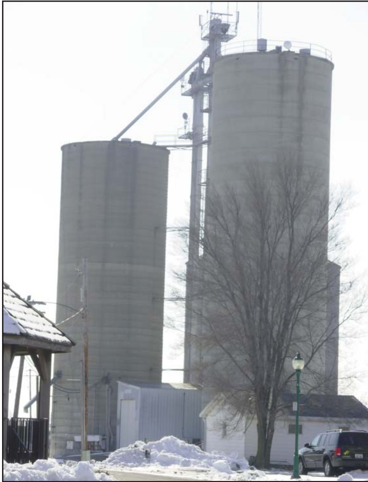
Prairie Central Cooperative grain elevators
