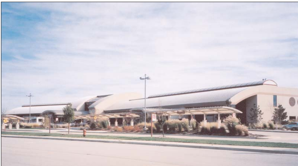
Central Illinois Regional Airport terminal
