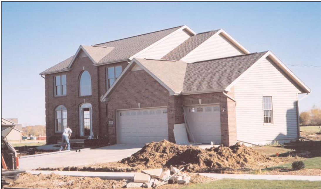
New construction in Fox Creek subdivision
