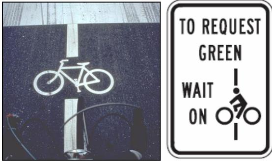
Figure 2.12. Signal activation marking and sign.
